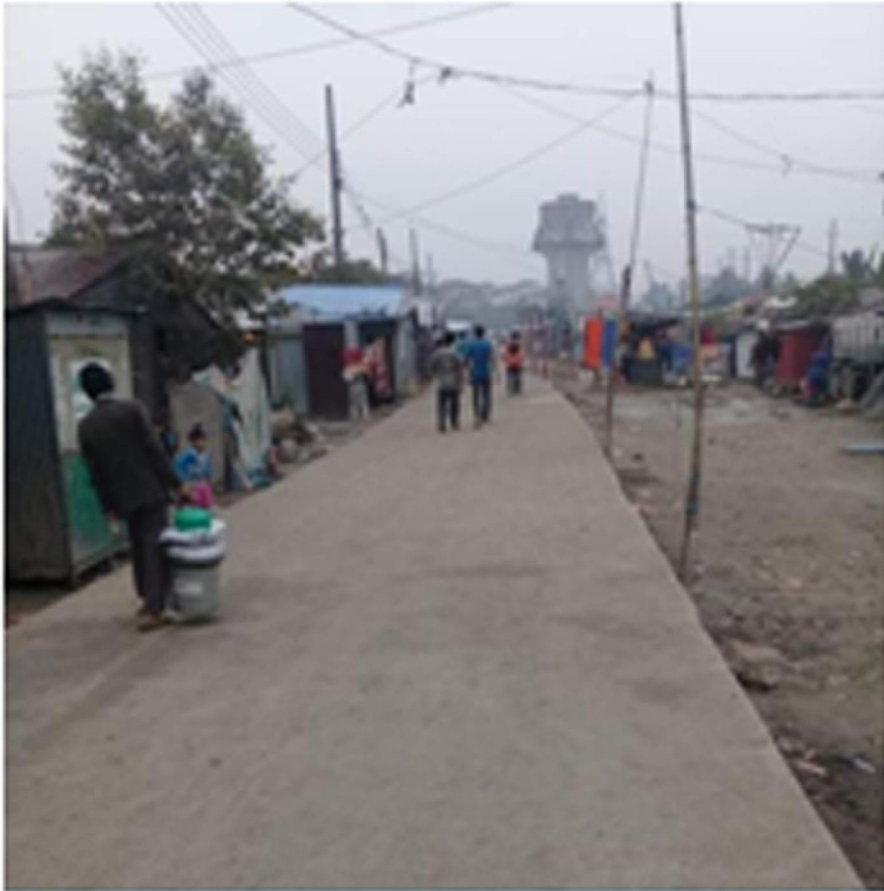
The newly constructed road of block-P
