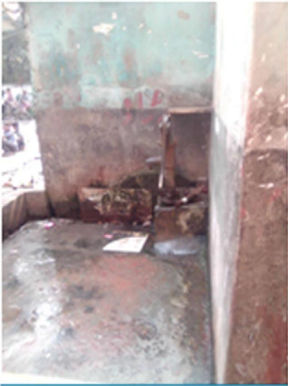
Tube-well adjacent to the cubicles
